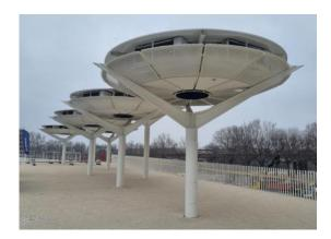
In addition to extracting pollution from vast volumes of air, these AEROPHILTRES offer several other advantages: they consume very little energy (1kW, equivalent to a refrigerator), require minimal maintenance (annual cleaning is sufficient), and serve as shading during the day and public lighting in the evening.
